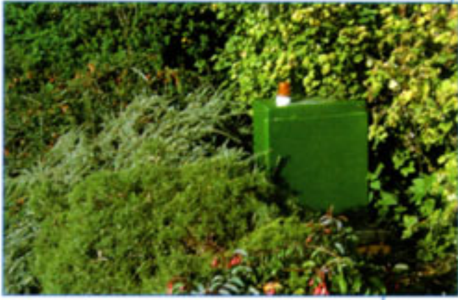
Existing septic tank refurbishment
