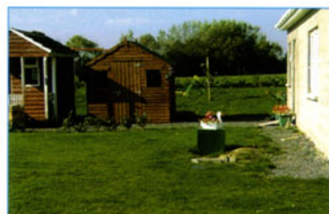
Single house sewage treatment plant for new house
